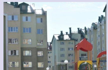
HOUSE RESOURCE CONSUMPTION METERING
