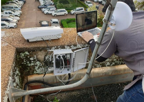
Picture 44. Installation of hardware at KCCA Library & Information Centre
