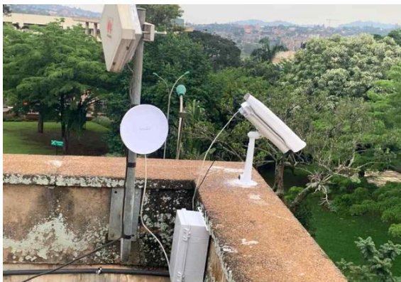
Picture 46. Finished installation of hardware at KCCA Library & Information Centre
